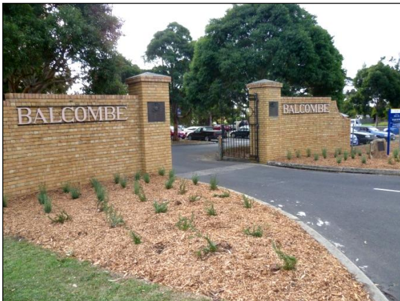
Balcombe Camp Gate – built by the Apprentices as a memorial to the 1 st Div US Marines
